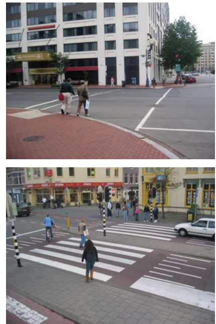
Figure 16: Existing crosswalk (above) and an example of ladder crosswalk with underlying red paint for added visibility (below).
