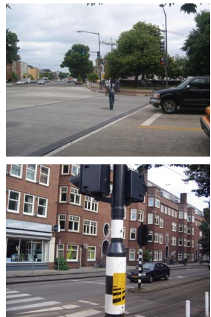
Figure 17: Existing setback of crosswalk (above) and an example of increase setback creating further separation between vehicles and pedestrians (below).
